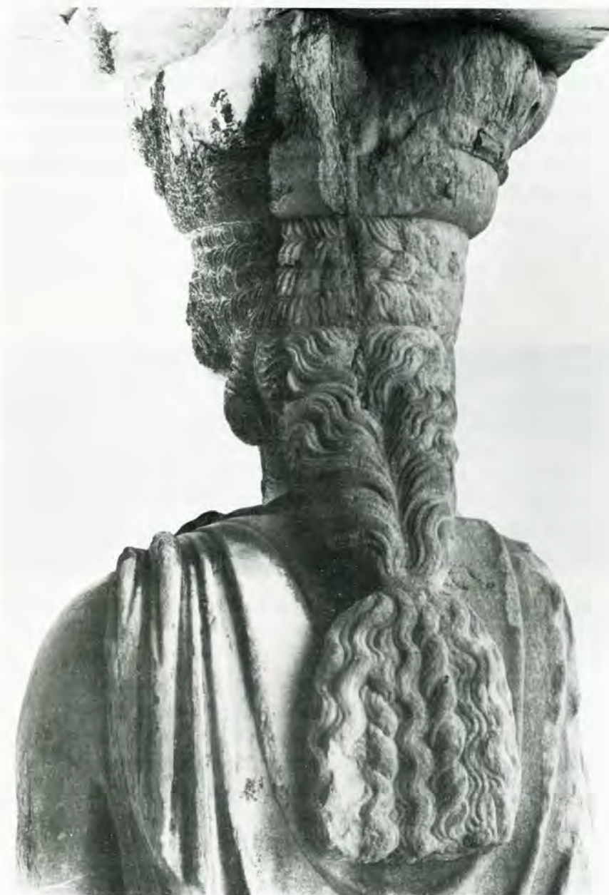
Fig. 4b. Sulphation on the back of a Caryatid. Rear surface protected from rainwater.
