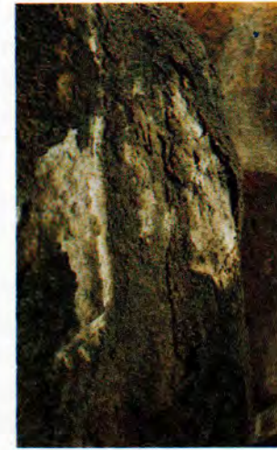
Fig. 29. Disintegration of the marble in conjunction with deposits of soot and the formation of black crust.
