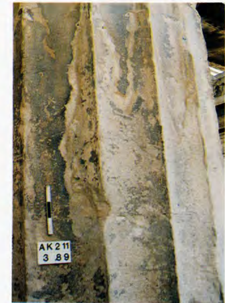
Fig. 40. After the reattachment of the delamination. Parthenon A.K. 2.11.
