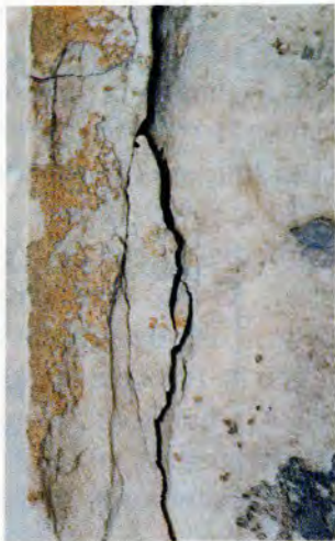
Fig. 27. Delamination. Detail from a Parthenon column.
