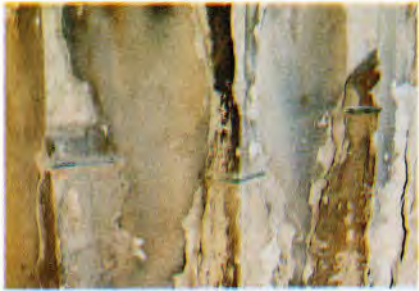
Fig. 37. Detail from previous consolidation intervention in 1922-1933 with Meyer cement and copper rivets. Parthenon A.K. 2.11.
