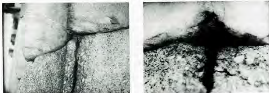
Fig. 2, 3. Successive steps in the cracking of concrete and marble owing to corrosion of the steel reinforcement. Detail from Balanos' restoration of a column on the Parthenon.
