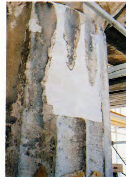
Fig. 39. The delaminated area after cleaning of the broken surface. A.K. 2.11.
