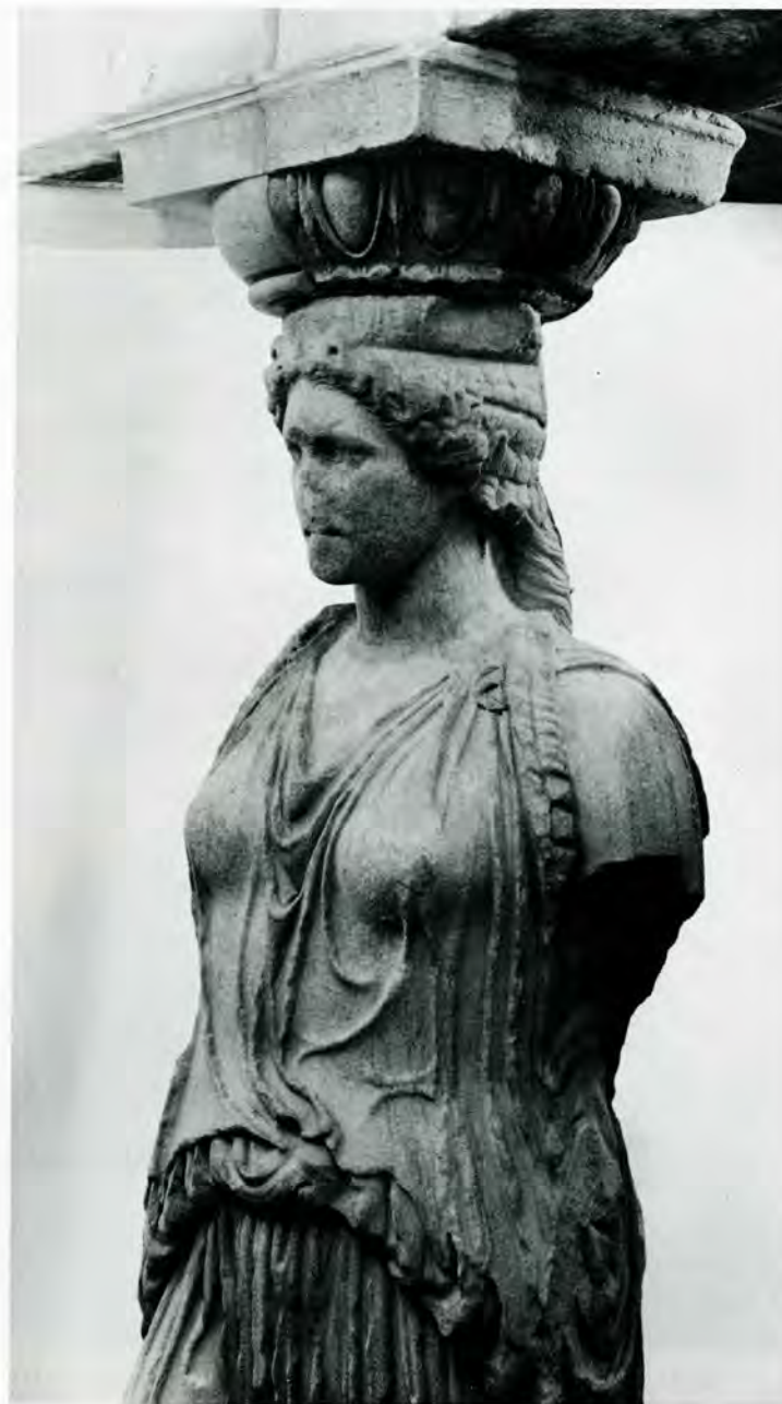
Fig. 4a. View of a Caryatid showing the acid attack by acid rain on the front.
