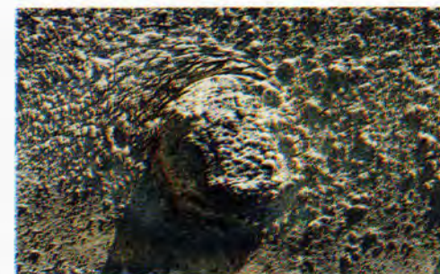
Fig. 33. Black dendritic crust on a Parthenon mutule..
