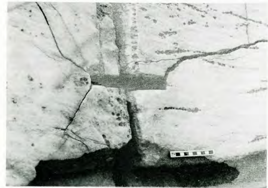
Fig. 1. Cracking of marble due to expansion of the steel junctions.
