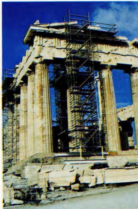
Fig. 47 View of scaffolding on east side of Parthenon.
