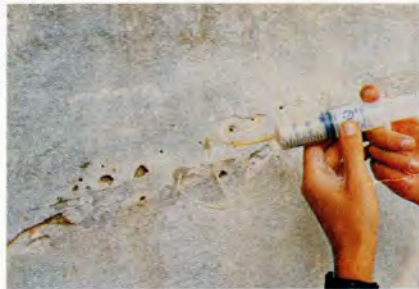
Fig. 41. Injection grouting of internal cavities. Propylaea. B-Δ.0.6.
