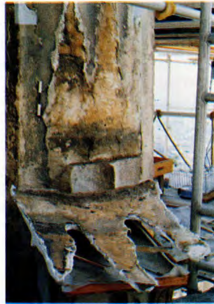
Fig. 38. Same region as shown in Fig. 37, after the delaminated piece has been detached. Parthenon A.K. 2.11.
