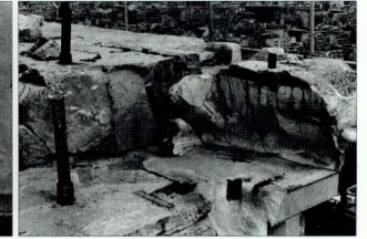
9-10. 金属部件（如夹子和榫钉）膨胀所导致的破裂。 9-10. Fracturing resulting from the swelling of metal components (clamps, dowels).
