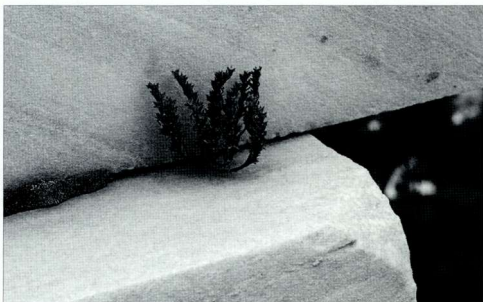
11-12. 帕特农神庙南柱廊的柱头和楣梁之间的鸽粪和寄生植物。 11-12. Pigeon droppings and parasitic plant growth between the column capital and the architrave of the south colonnade of the Parthenon.
