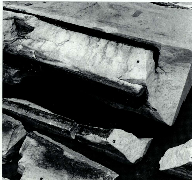
8. 早期修复时使用的铁夹生锈膨胀，导致神庙上楣柱破裂。 8. Fracturing of the cornice caused by the swelling of rusted iron clamps introduced in earlier restoration.
