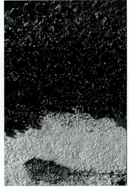
6. 帕特农神庙楣梁下方的大理石水晶面已失去粘着力，并受碳化作用和灰尘的影响，形成了一个黑痂。 6. Detail of the lower surface of a Parthenon architrave where the marble crystals have lost their cohesion and a dark crust has been formed, caused by carbonization and dust.
