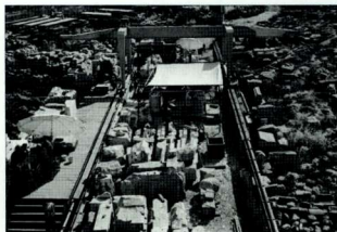
120-122. 卫城工地现场东部。修复工程正在进行之中，采用桥式起重机拆卸和组装建筑构件（2002年）。 120-122. The area east of the Propylaea work-site. Work in process and architectural members that have been disassembled and organised, within range of the bridge-crane (2002).
