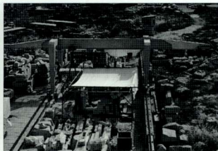
120-122. 卫城工地现场东部。修复工程正在进行之中，采用桥式起重机拆卸和组装建筑构件（2002年）。 120-122. The area east of the Propylaea work-site. Work in process and architectural members that have been disassembled and organised, within range of the bridge-crane (2002).
