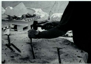
64. 利用机械手段去除铁制加固件。 64. Removal of iron reinforcements by mechanical means.
