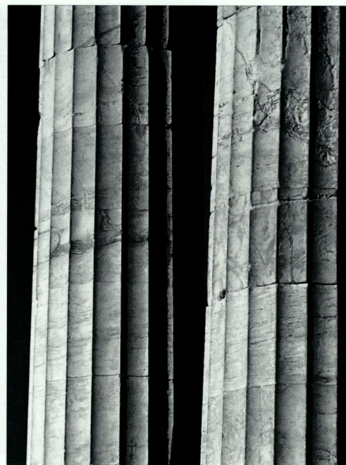
76. 南侧柱身细部。 76. Detail of column shafts of the south side.
