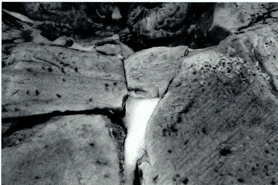
13. 冰冻导致裂缝加宽。 13. Crack widened by freezing.
