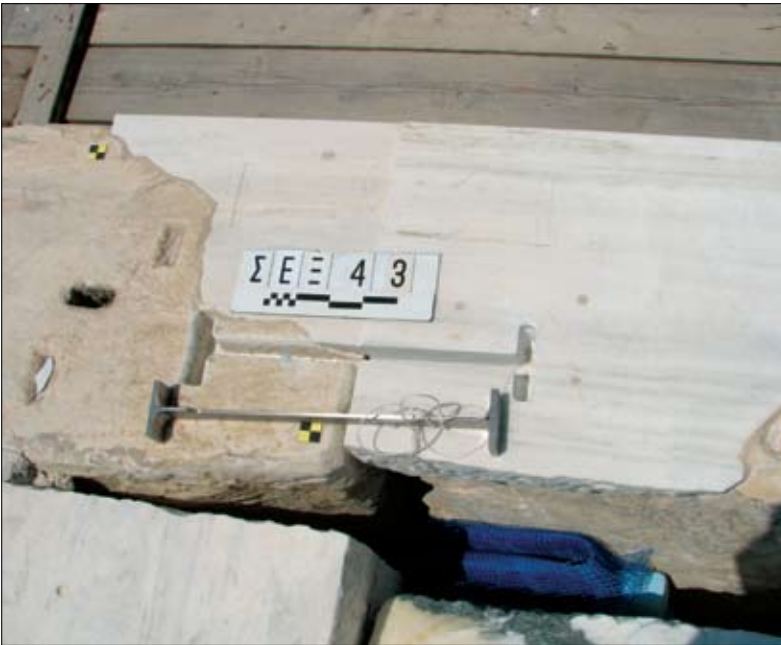
12. Setting a double-T clamp of titanium for joining two architrave blocks in the north side of the Parthenon.
