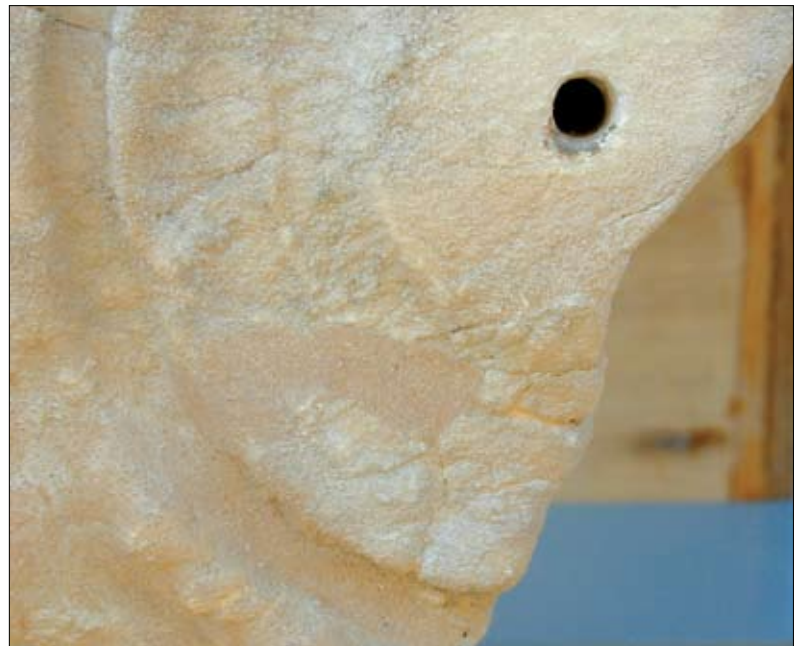
13a-b. Column capital of the east porch of the Erechtheion. Condition of the surface before and after conservation.
