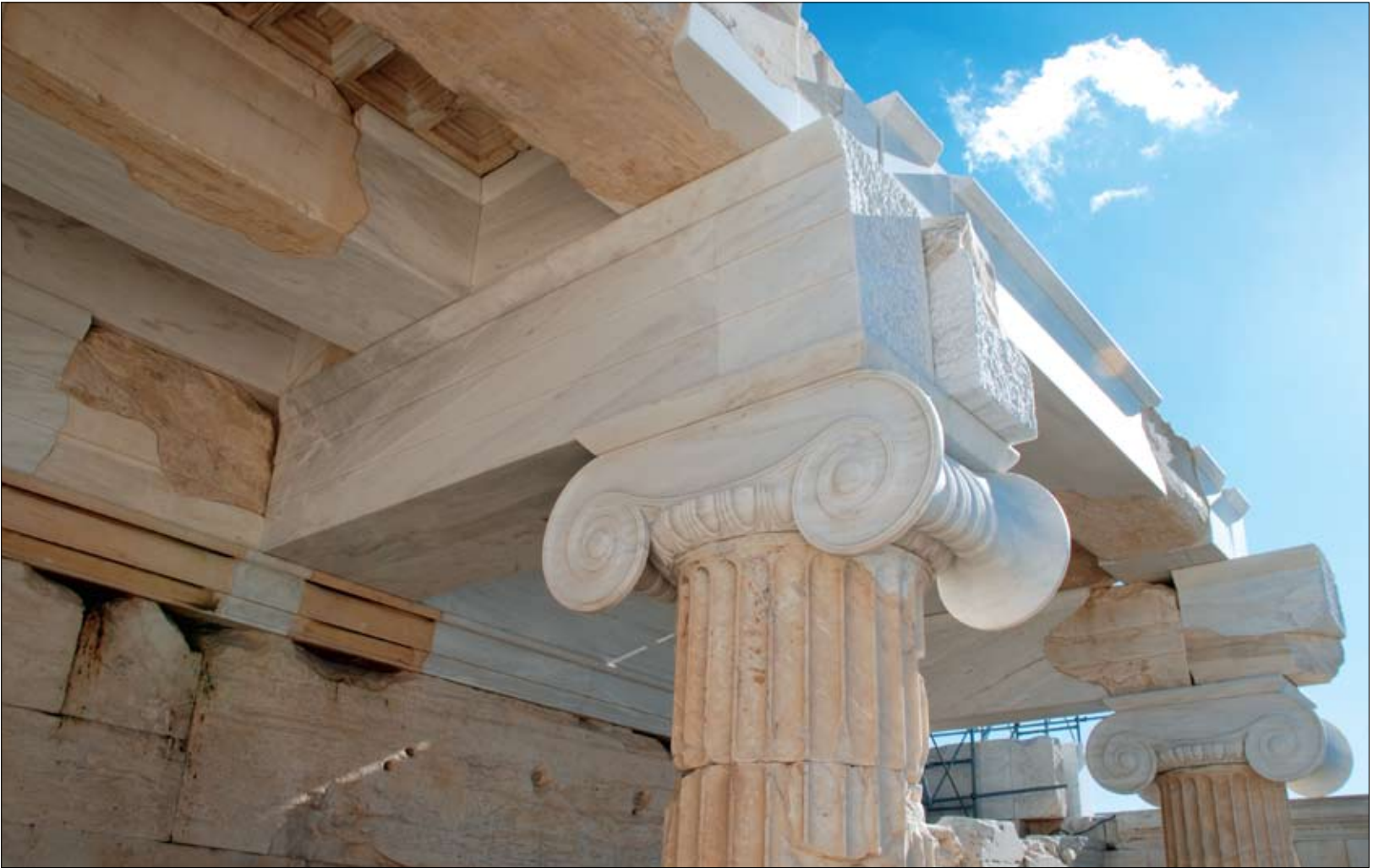
56. Propylaea. The ceiling of the west hall after anastelosis. Visible are the two copies of the Ionic column capitals. View from the northwest.
