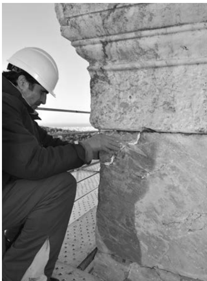
View from the E during works for the reattachment of a fragment of the monument's shaft. Photo P. Vlachouli, 2022
