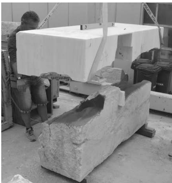
Adjustment of the new marble addition on the ancient block Δ.TA4.6. Photos V. Manidaki, 2022
