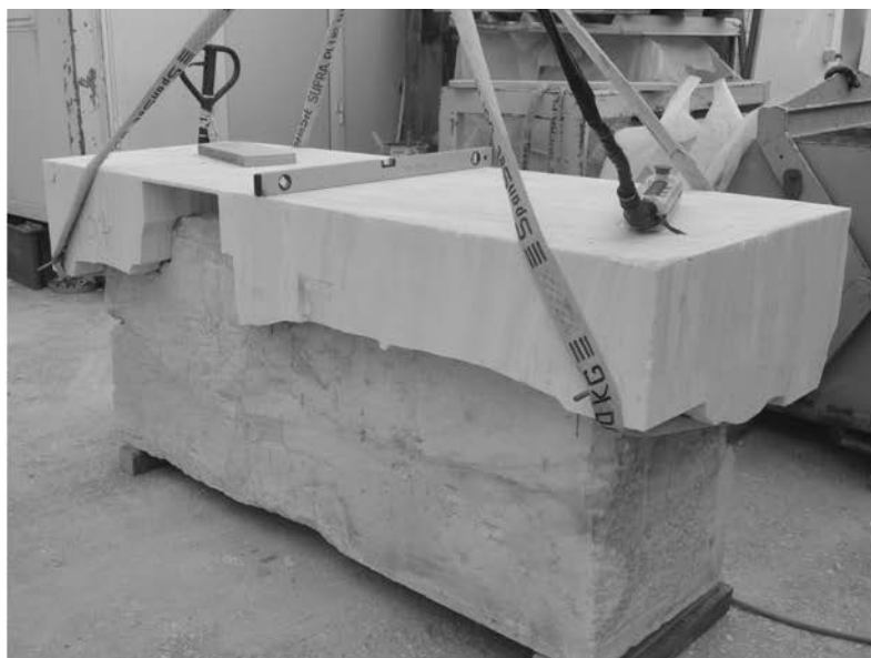
Adjustment of the new marble addition on the ancient block Δ.TA4.6. Photos V. Manidaki, 2022
