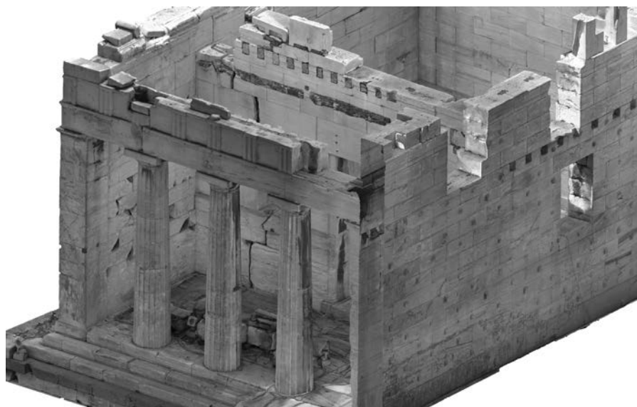
Photo-textured three-dimensional model of the north wing of the Propylaea. Study: "Production of three-dimensional model of the Propylaea north wing", 2021
