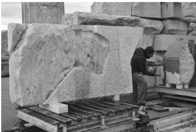
Elaborating a fragment for the orthostate of the south wall of the Parthenon cella. Photo R. Christodouloupoulou, 2022
