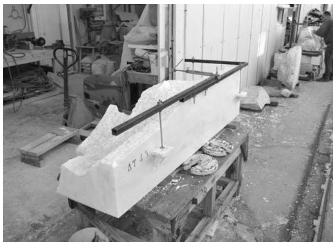
The traditional method of creating new marble additions with the use of a pointing device. Photos K. Skaris, 2020
