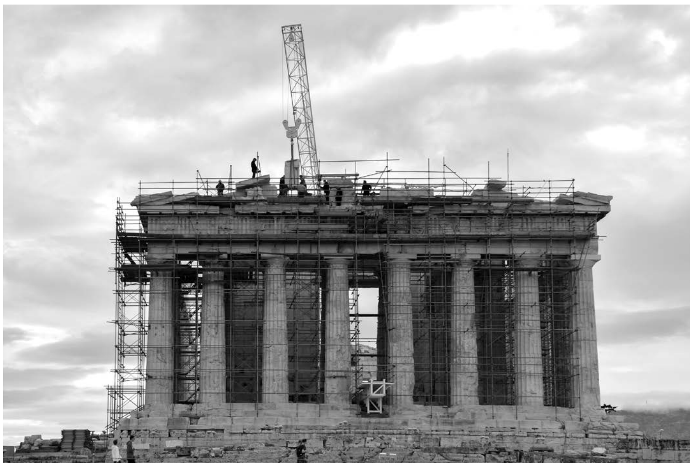
Trial positioning of an orthostate block in the Parthenon's west pediment. Photo K. Karanasos, 2021
