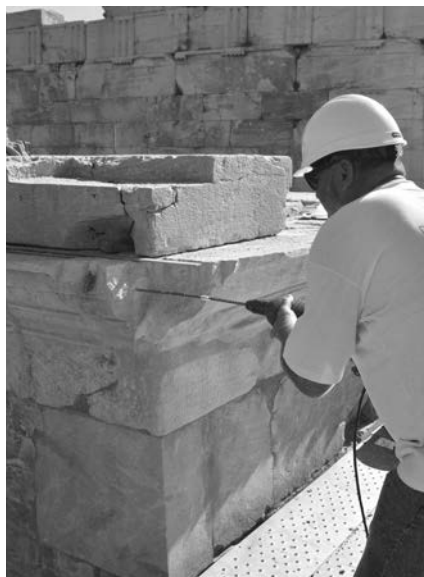
View from the SW during the consolidation of a stone of the monument's crown. Photo K. Karanasos, 2022
