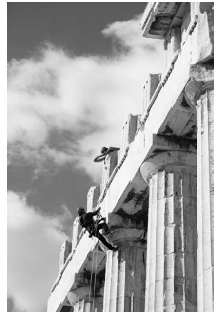
Clearing vegetation from the monuments, 2021
