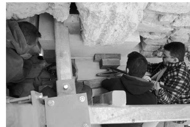
Placing a new block in the area B17. Photo K. Mamalougas, 2019
