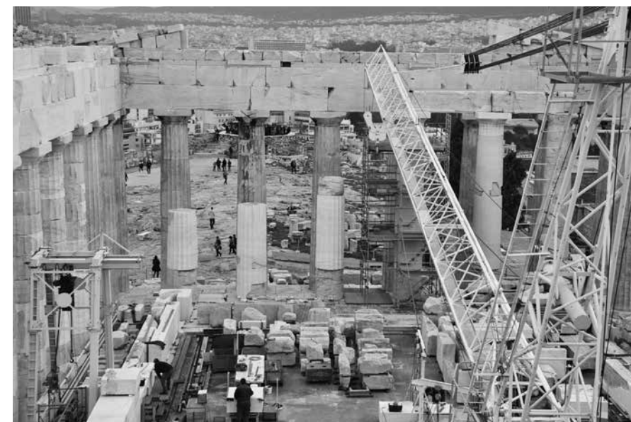
A view of the Pronaos from the west. We can see the first three from the north columns where the carving of the flutes has been completed. Photo T. Souvlakis, 2020
