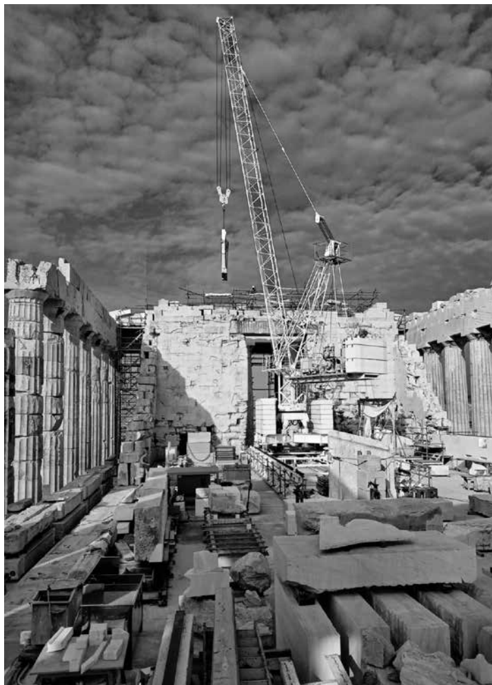
The crane POTAİN MR90 at the Parthenon. Photo G. Kehagias, 2020
