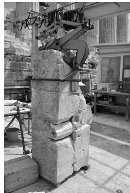
Works of structurally reconstructing a block (Δ.TA.3.3) of the retaining wall of the west Parthenon pediment. Photo K. Skaris, 2020
