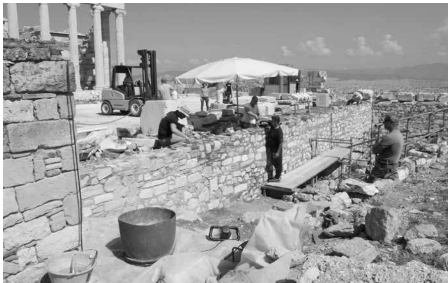
Restoration works on the retaining walls in the area of the Mycenaean ascent. Photo Ch. Pinatsi, 2019
