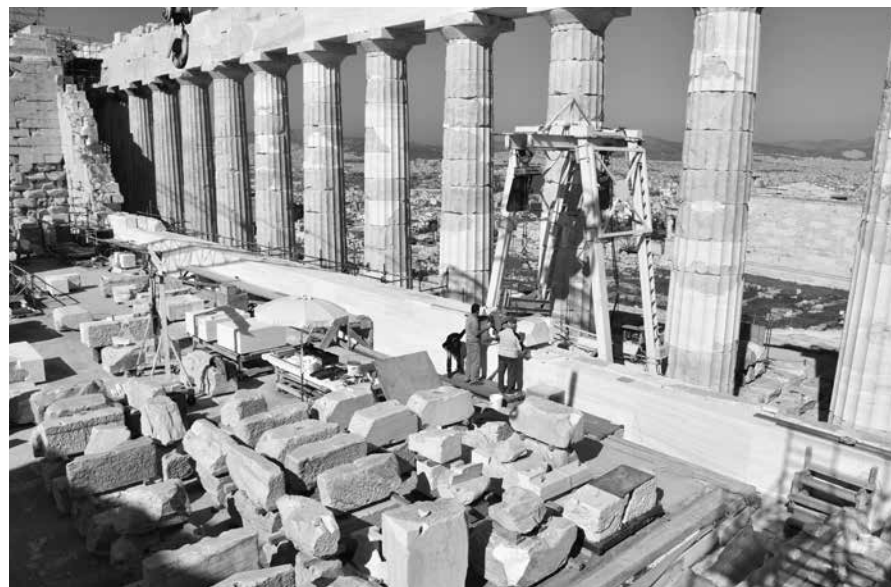
Restoration works on the first row of the north wall of the Parthenon cella. Photo T. Souvlakis, 2020
