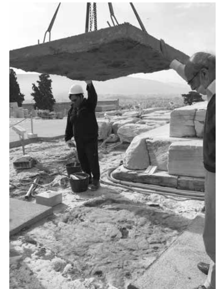
Removing samples to test out the adhesion of the material on the rock and confirm the intervention reversibility. Photo T. Souvlakis, 2021
