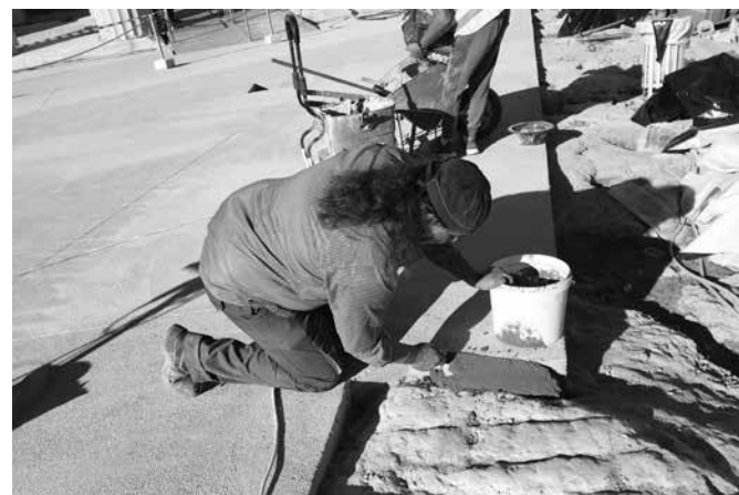
Works of laying the walkways. Top left: covering the rock with gravel and placing pipes for cable routing. Top right: laying concrete on the protective film. Bottom left: laying concrete in an area where metal reinforcement is incorporated. Bottom right: filling concrete to even the contact of the walkways with the natural rock. Photos V. Manidaki, 2020.
