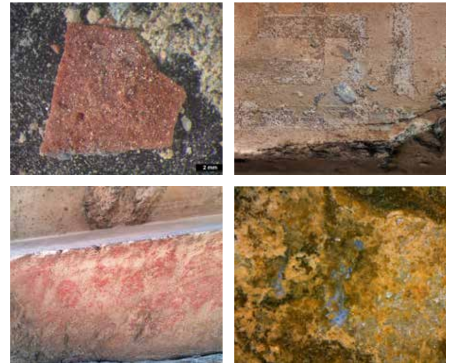
Cornice blocks of the west side of the Parthenon. Top left: The 4 th west cornice block: red pigment from the via. Photo from the stereomicroscope. Top right: The 21 st west cornice block: the meander grid on the taenia. Bottom left: The 11 th west cornice block: a red pigment layer at the bottom of the taenia. Bottom, right: The 14 th cornice block: blue colour on the meander under a layer of orange-brown patina.
