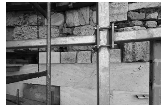
The west edge of the intervention area after placing new blocks Photo K. Mamalougas, 2019
