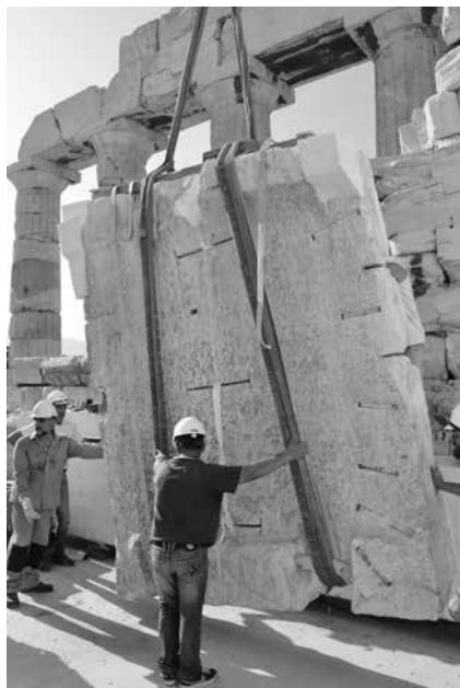
The central orthostate of the tympanum of the west Parthenon pediment during the restoration works. Photo V. Manidaki, 2020
