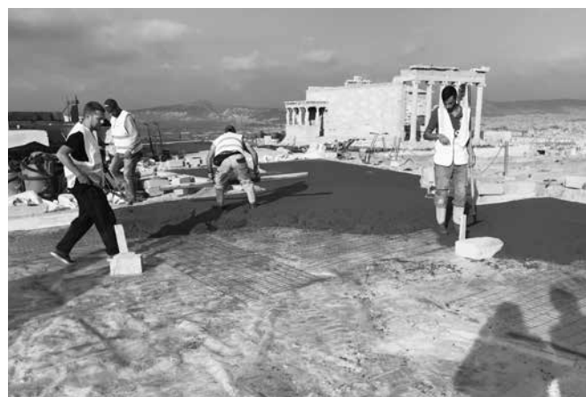
Works of laying the walkways. Top left: covering the rock with gravel and placing pipes for cable routing. Top right: laying concrete on the protective film. Bottom left: laying concrete in an area where metal reinforcement is incorporated. Bottom right: filling concrete to even the contact of the walkways with the natural rock. Photos V. Manidaki, 2020.
