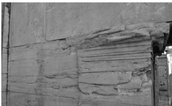
Top, left: The Parthenon: a block from the retaining wall of the west pediment (Δ.TA.I.5) before the conservation works. Top, right: the same block after conservation. Photo A. Panou, 2020. Bottom, left: The Propylaia: a block of the portal wall of the north wing (B.Θ.I.7) before the conservation interventions. Bottom, right: the same block after conservation. Photo P. Vlachouli, 2020
