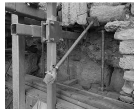
Temporary shoring of the masonry during the dismantling period. Photo K. Mamalougas, 2019
