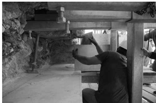
Placing a new block on the area B17 of the north wall. Photo K. Mamalougas, 2019
